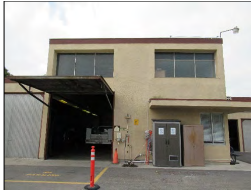
Vehicle Maintenance Shop, north elevation, center projection, view south (LSA 2021)
