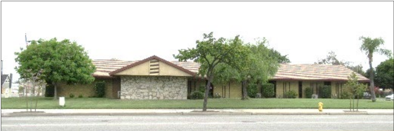
Administration Building, south elevation, view north (LSA 2021)
