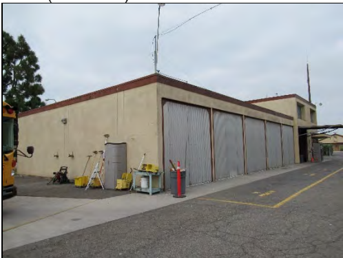
Vehicle Maintenance Shop, north elevation, view southwest (LSA 2021)
