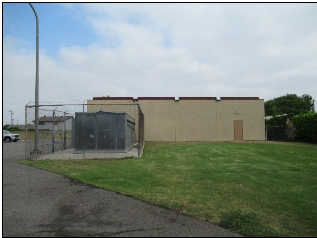
Warehouse, south elevation, view north (LSA 2021)
