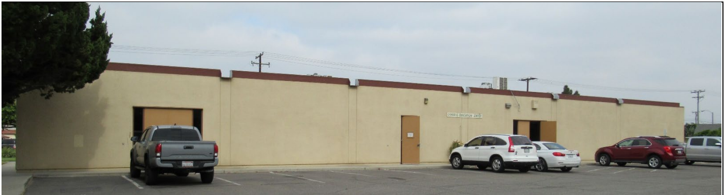
Educational Center, east elevation, view west (LSA 2021)
