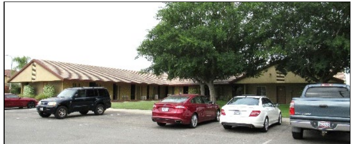
Administration Building, north elevation (left) and east elevation (right), view southwest (LSA 2021)
