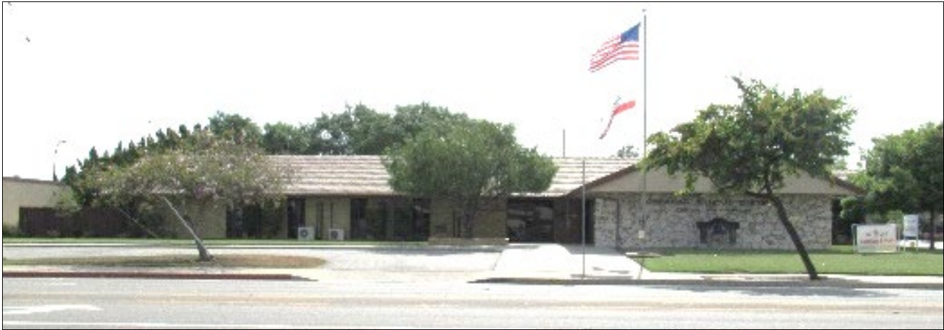
Administration Building, west elevation, view east (LSA 2021)
