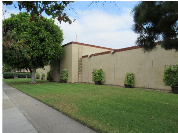
Figure 16: Vehicle Maintenance Shop, south elevation, view northwest (LSA 2021)
