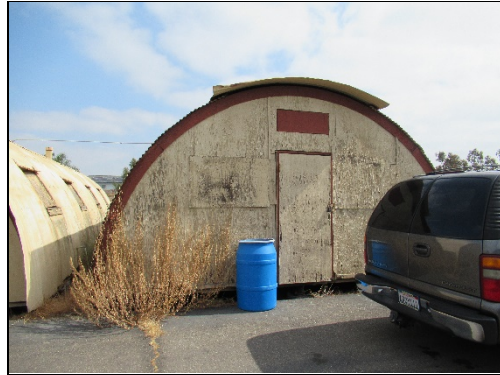
Quonset Hut, south elevation, view north (LSA 2021)
