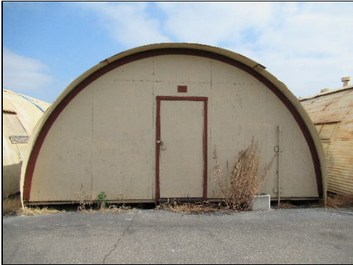
Quonset Hut, south elevation, view north (LSA 2021)
