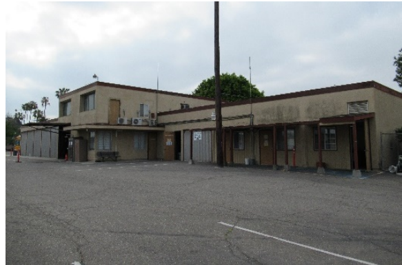
Figure 14: Vehicle Maintenance Shop, north elevation, view southeast (LSA 2021)
