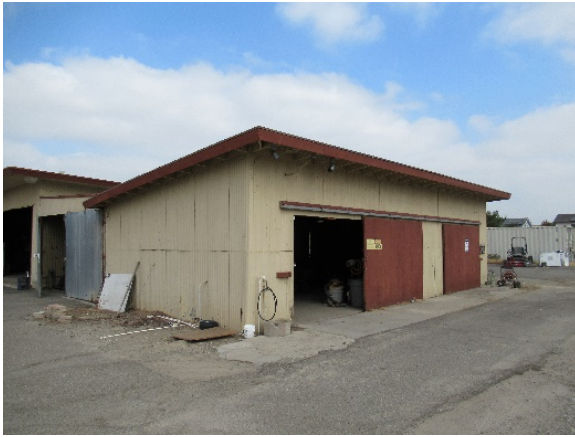
Figure 19: Maintenance Shop and Equipment Storage Shed, south elevation (left) and east elevation (right), view northwest (LSA 2021)
