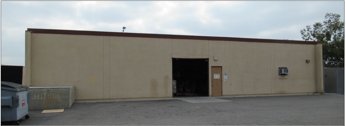
Warehouse, west elevation, view east (LSA 2021)
