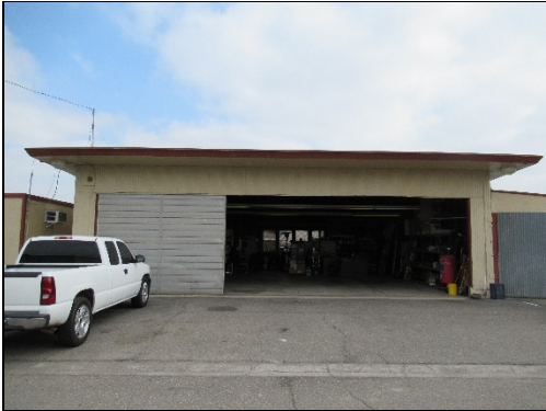
Maintenance Shop, south elevation, view north (LSA 2021)
