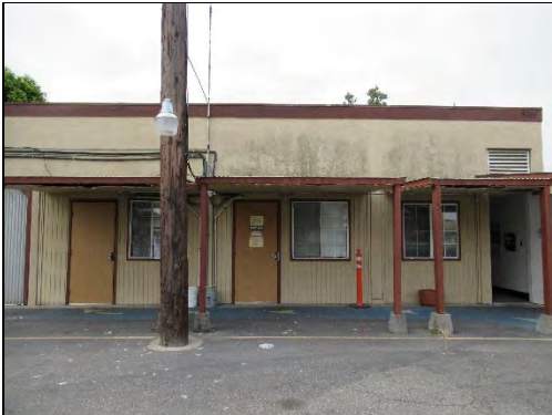
Vehicle Maintenance Shop, north elevation, west section, view south (LSA 2021)
