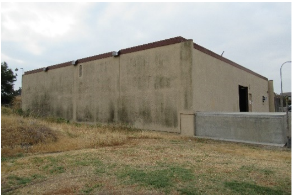
Figure 12: Warehouse, north elevation (left) and west elevation (right), view southeast (LSA 2021)
