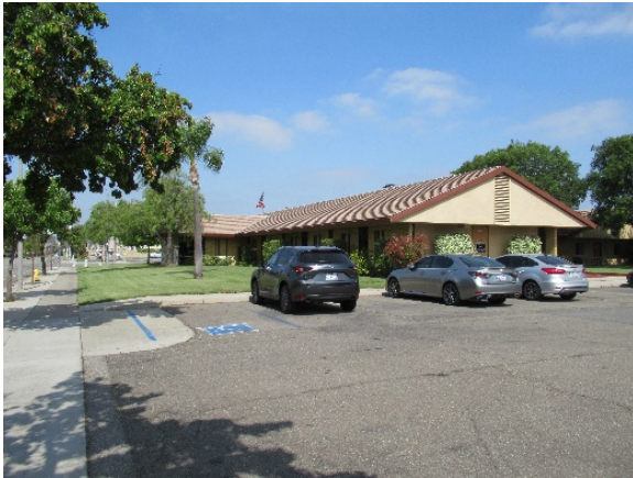
Figure 7: Administration Building, east elevation (right) and south elevation (left), view northwest (LSA 2021)
