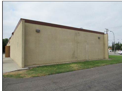
Educational Center, north elevation, view south (LSA 2021)
