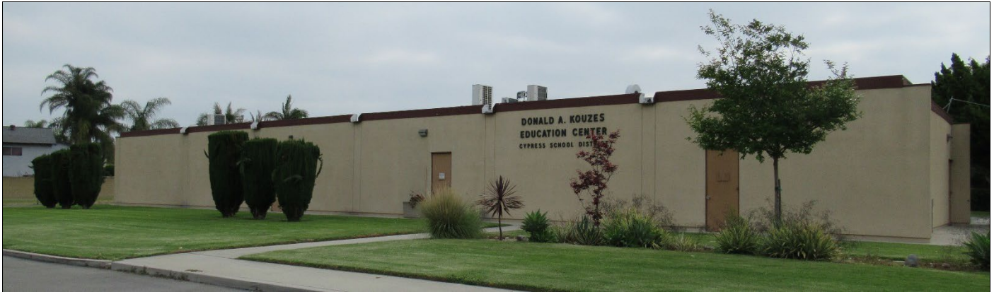
Educational Center, west elevation, view northeast (LSA 2021)
