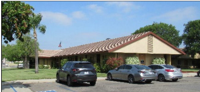
Administration Building, east elevation (right) and south elevation (left), view northwest (LSA 2021)
