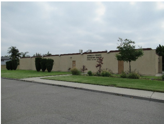
Figure 9: Educational Center, west elevation, view northeast (LSA 2021)
