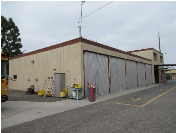
Figure 15: Vehicle Maintenance Shop, east elevation (left) and north elevation (right), view southwest (LSA 2021)
