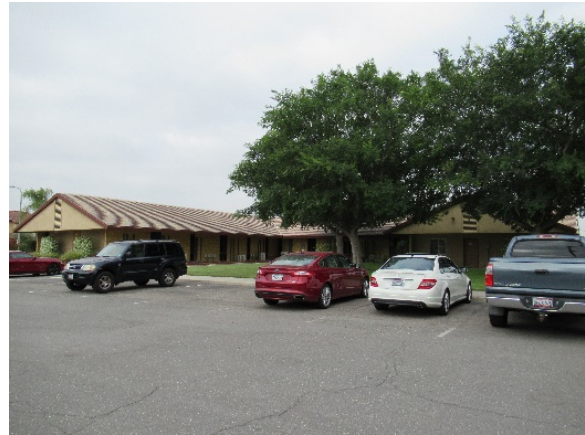
Figure 8: Administration Building, north elevation (left) and east elevation (right), view southwest (LSA 2021)
