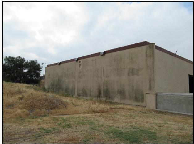
Warehouse, north elevation, view southeast (LSA 2021)
