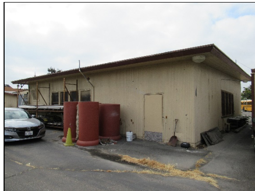
Maintenance Shop, north (left) and west (right) elevations, view southeast (LSA 2021)
