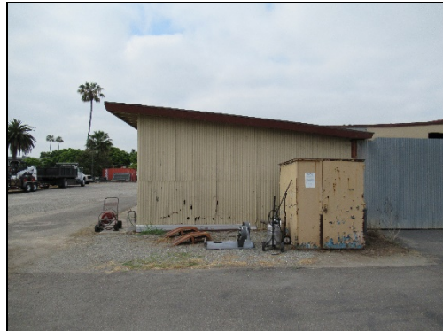
Equipment Storage Shed, north elevation, view south (LSA 2021)
