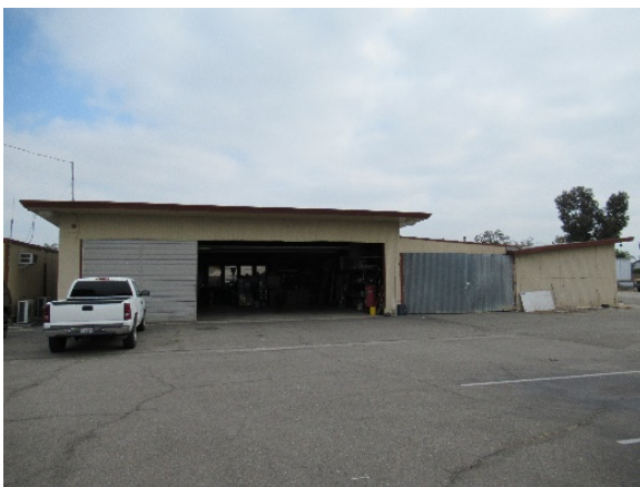
Figure 17: Maintenance Shop and Equipment Storage Shed, south elevation, view north (LSA 2021)
