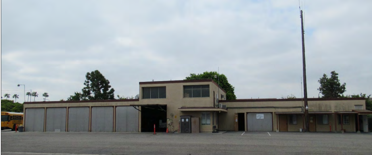
Vehicle Maintenance Shop, north elevation, view south (LSA 2021)
