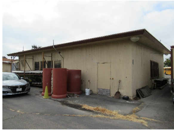
Figure 20: Maintenance Shop and Equipment Storage Shed, north elevation (left) and west elevation (right), view southeast (LSA 2021)
