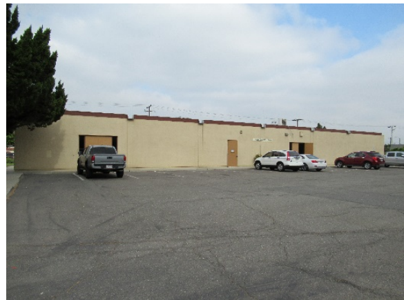
Figure 10: Educational Center, east elevation, view west (LSA 2021)
