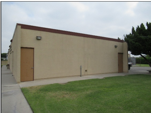
Educational Center, south elevation, view north (LSA 2021)
