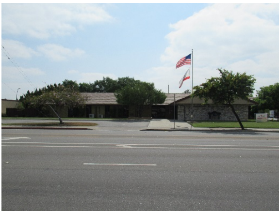
Figure 5: Administration Building, west elevation, view east (LSA 2021)
