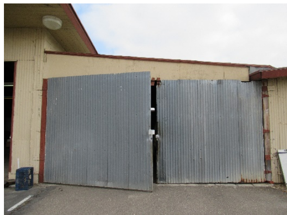
Figure 18: Maintenance Shop and Equipment Storage Shed, south elevation, view north (LSA 2021)
