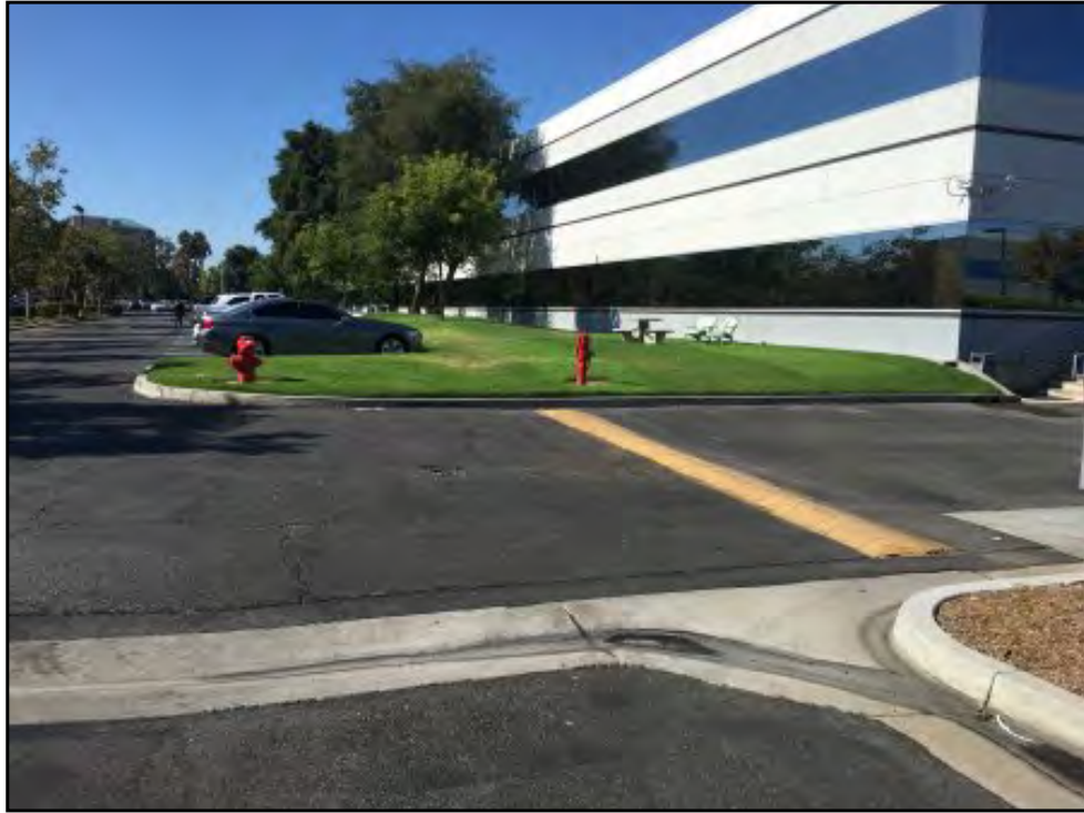
Eastern side of building
