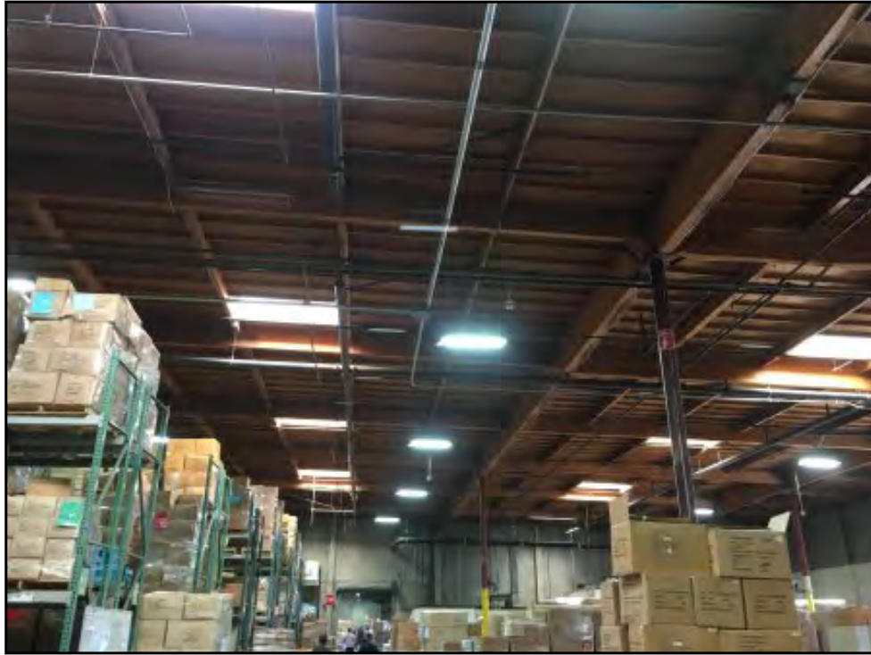
Hybrid Apparel warehouse ceiling
