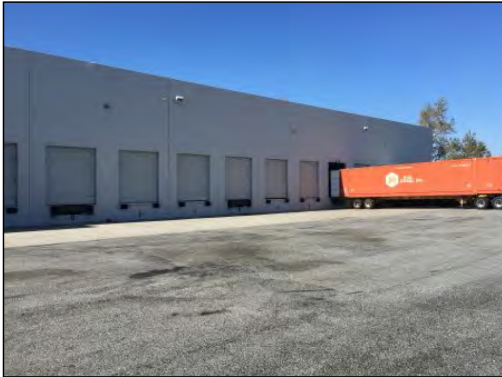
Additional loading bays on north side of building
