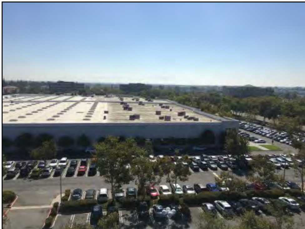
View of rooftop from distance
