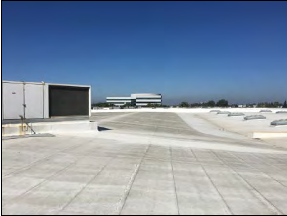
Western view of roof
