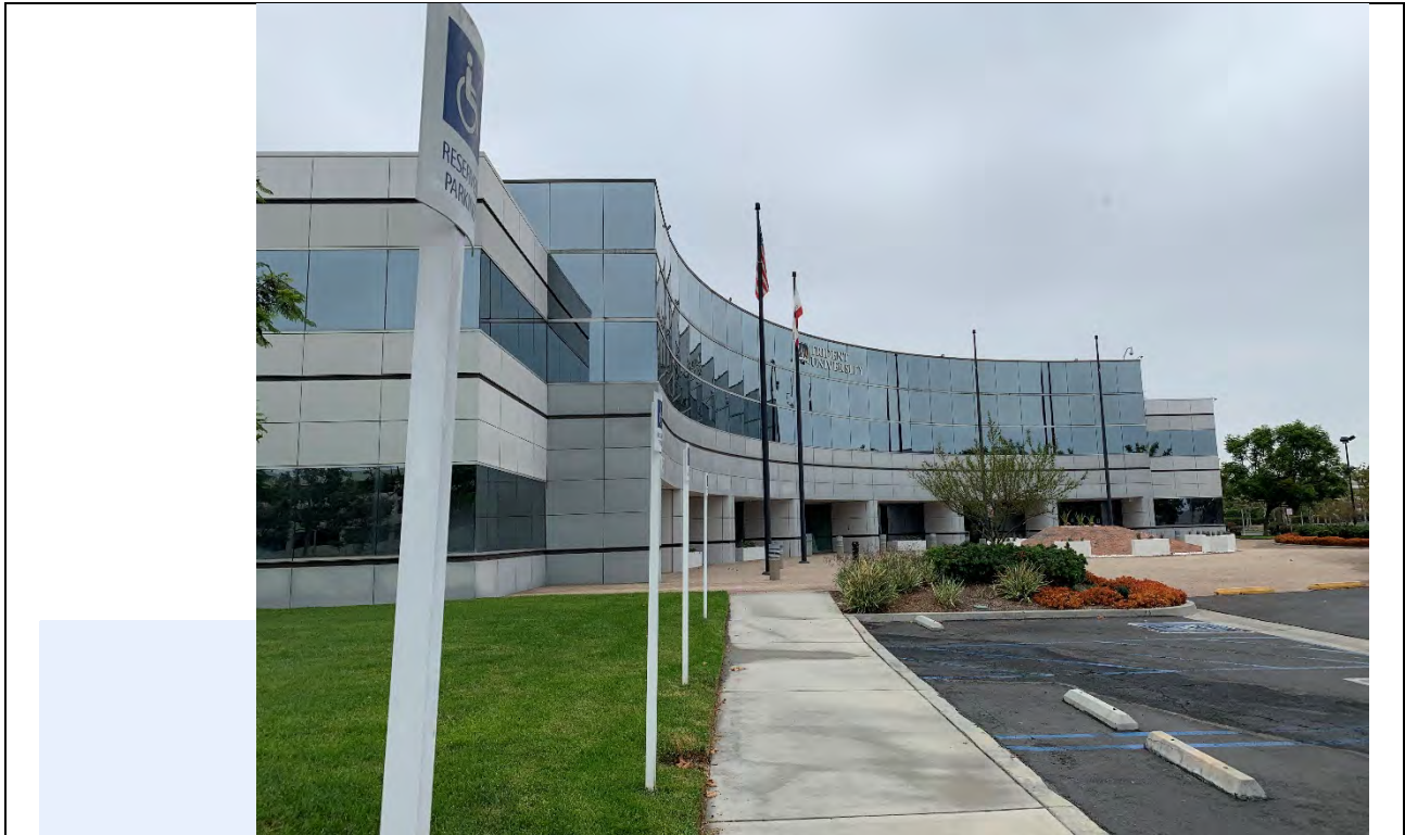
Photo #1 View of the 5757 Plaza Drive building exterior.
