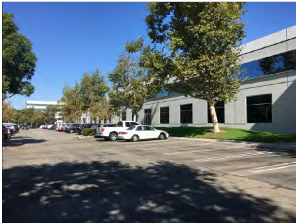
Additional view of southern portion of building
