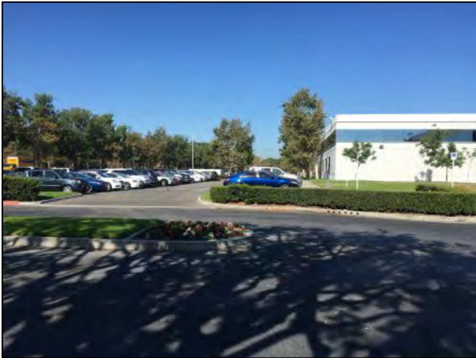
Western view of southern portion of building
