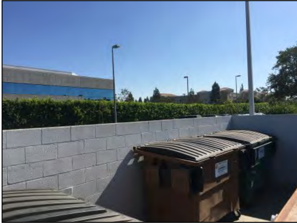
Dumpsters within enclosure
