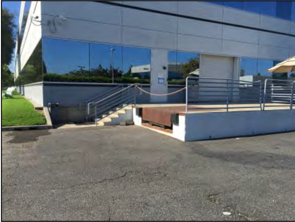
Northeastern portion of building
