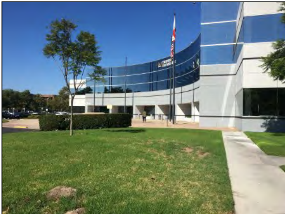
Main entrance of building
