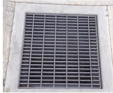
Grates should be kept clear and clean.
