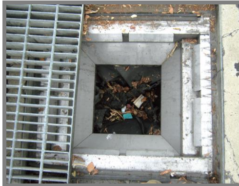
Drainage Insert (Area Inlet)
