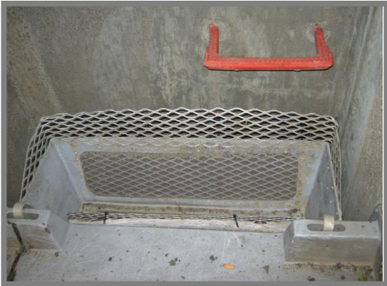
Drainage Insert (Curb Inlet)
