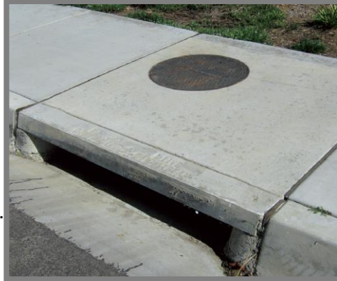
Drainage Insert (Curb Inlet)
