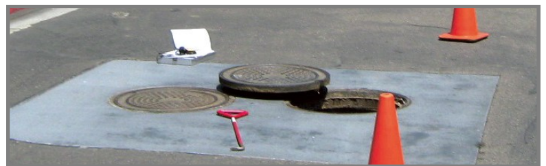
Units typically accessed through 2 or more adjacent manholes
